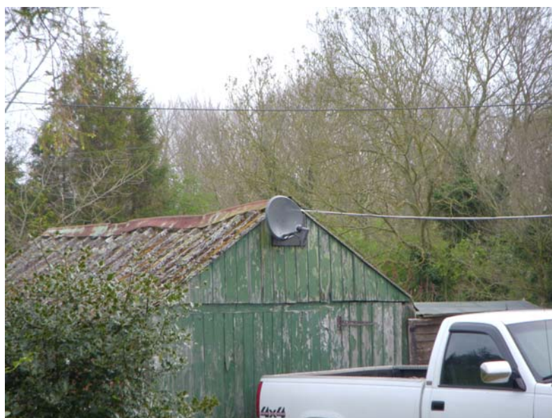
Satellite dish located on an outbuilding to avoid compromising the historic structure
