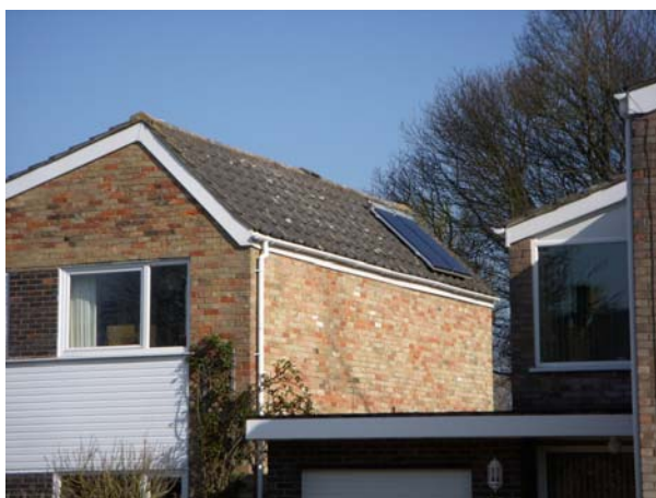
Discretely located solar panel on a side elevation of a 20 th century house in the Fulbourn Conservation Area
