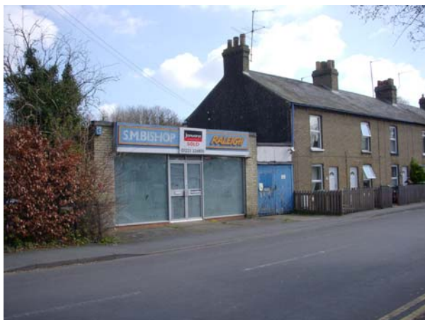
Bishop's Cycles in Histon Conservation Area, where consent has been granted for its demolition but the demolition cannot commence until consent has been granted for the redevelopment of the site
